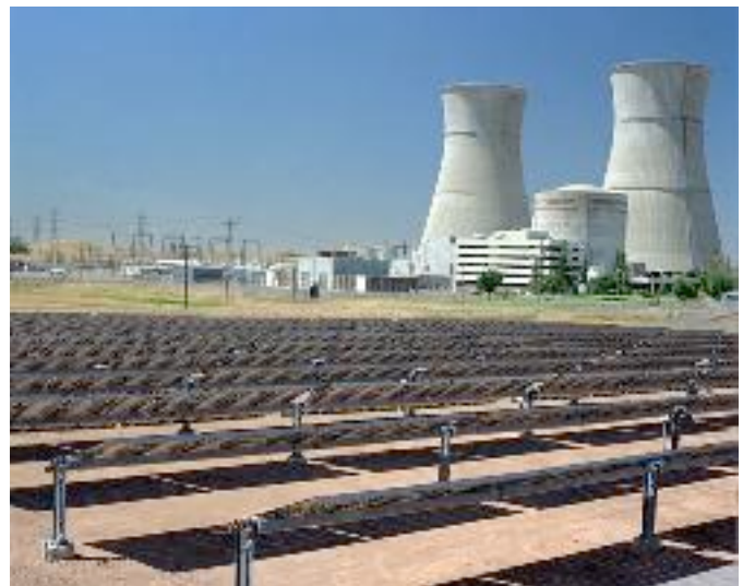
Rancho Seco nuclear reactor near Sacramento, closed by a democratic vote of the citizens, one megawatt solar electric installed next to the reactor
